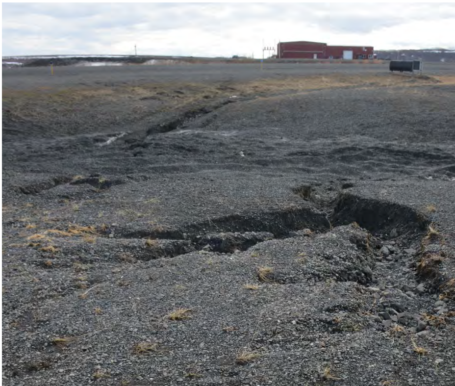
Graphic 4: Current Drainage Deficiencies on Runway 17/35
